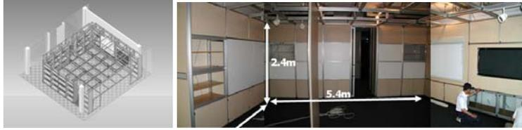
**Fig. 2.** Structure of the Box-in-the-Box
